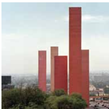
Torres de la Ciudad Satélite (Towers of Satellite City), Mexico City, 1957. Photo : Kim Zwarts, 02.1988
